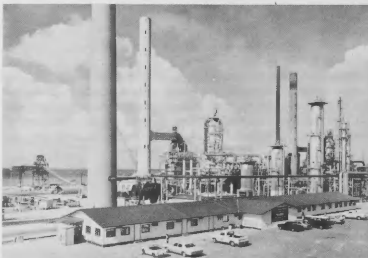
View of new HDS-II facilities built on reclaimed land.
